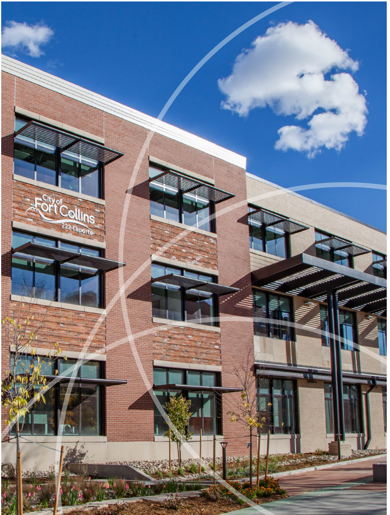
This municipal building was the first LEED v4 Platinum building constructed in Colorado.
